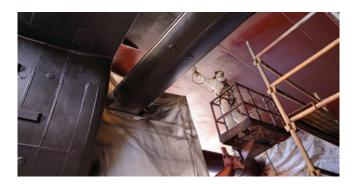
A patented self-polishing binder composition results in excellent film formation with high-volume solids (70%), making this technology ready for future legislation on lowering solvent emissions.
